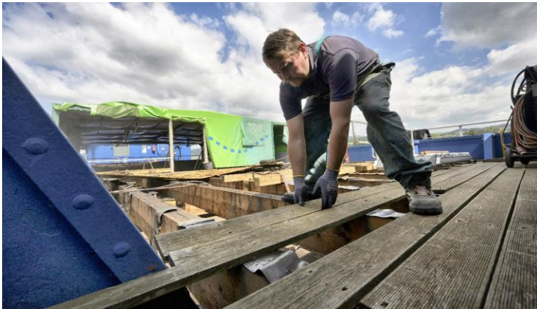
Figure 4: Dismantling of the ship's deck (© Zinner).
