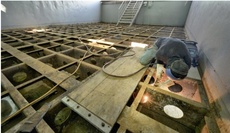
Figure 6: Renovation of the substructure under the cargo hold (© Zinner).
